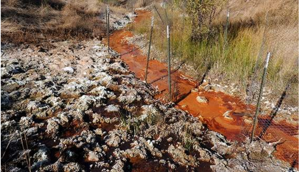
Crusty mineral formations cover rocks next to a creek flowing with discolored water below a landfill where 350,000 cubic yards of waste from a former mine are stored near Camanche Reservoir.
